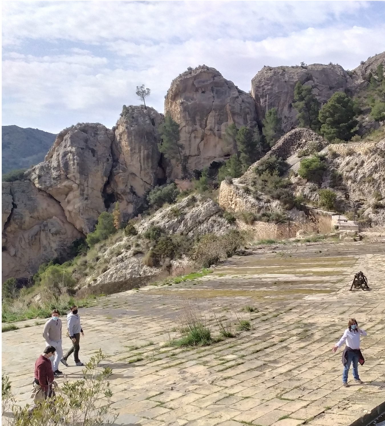
^ Fig. 2 Tibi dam on the Monnegre River in the province of Alicante, Spain. The site is revalorized as part of the “Blue Routes” tourist attraction and Monnegre Green Corridor strategy connecting diverse water-linked heritage sites (Source: Brigitt Albers, Bureau Vormgeving).
